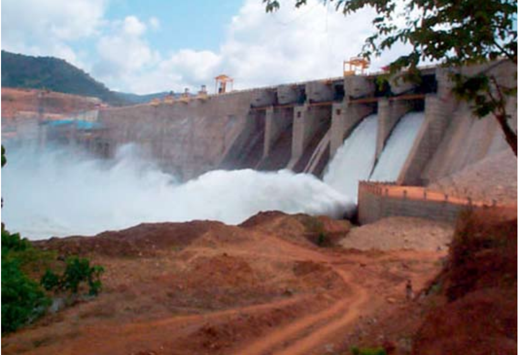
Geru Soppa Hydro Electric Project
