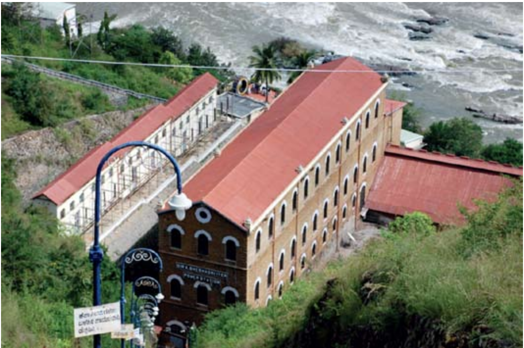
Sir K. Sheshadri Iyer Hydro Power Station, Shivasamudra Malavalli Taluk, Mandya District
